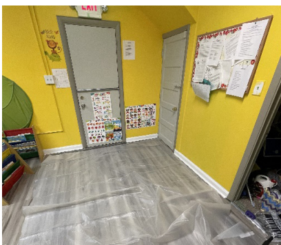
Prepping the work area for lead renovations
