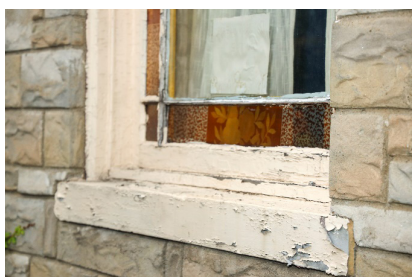
Peeling paint on exterior window was depositing on the ground where children enter the center.
